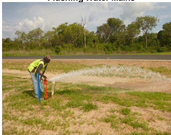
Flushing Water Mains
