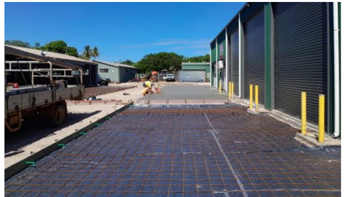
Workshop Concrete Access Works - LCRI Funding: May/June 2024
