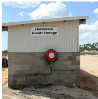
Purpose-built hazardous waste shed Pormpuraaw Aboriginal Shire, Sept. 2016
