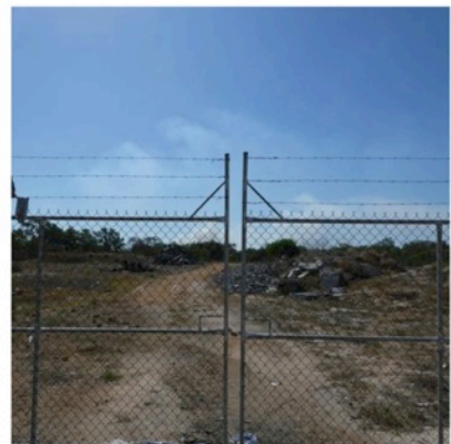
Compartmentalised landfill compound Pormpuraaw Aboriginal Shire, Sept. 2016
